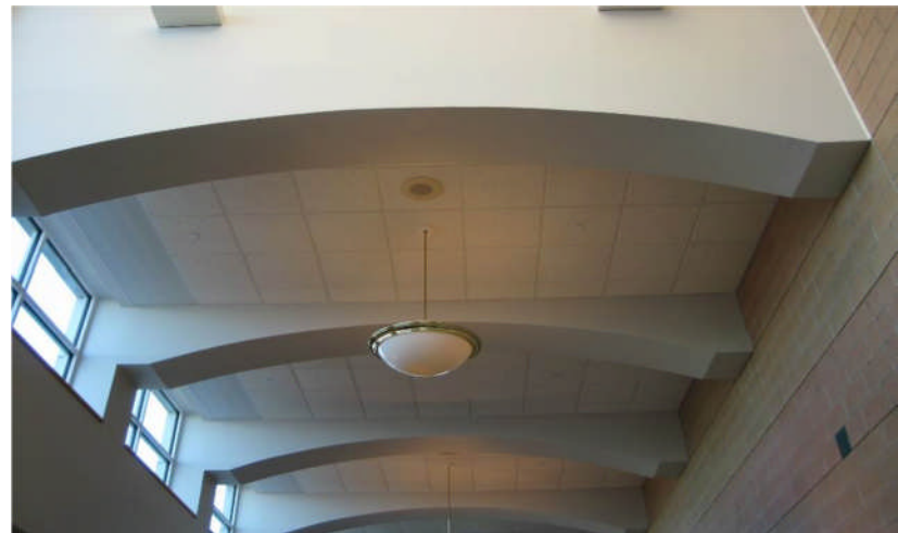
Health Education Building – Daylighting controls for the Atrium would save energy.
