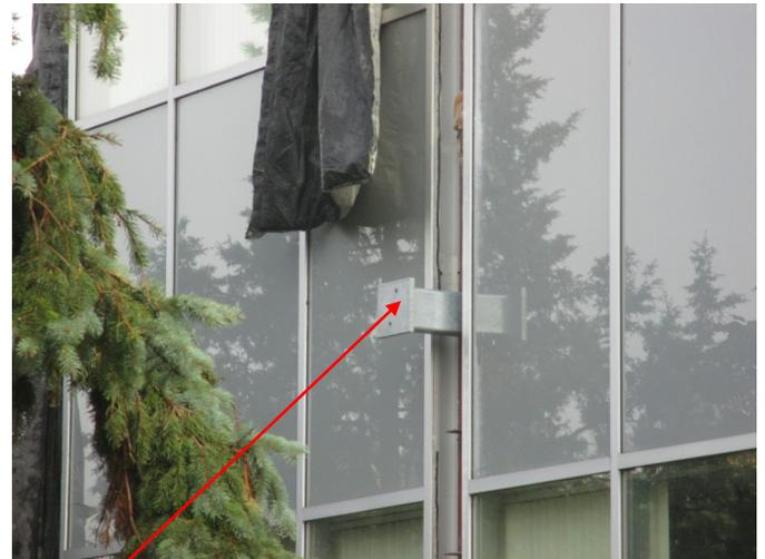
The top-left photo highlights the work being done on the south-west façade of the building. Here steel connectors are being welded to the building frame so the new metal screen veneer can be attached in front of the existing brick.
