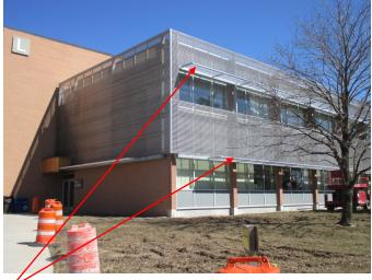
The top-left photo shows the progress of the installation of the horizontal portion of the new sunshade system on the south face of the existing building. Both the first and second floors are nearly complete.
