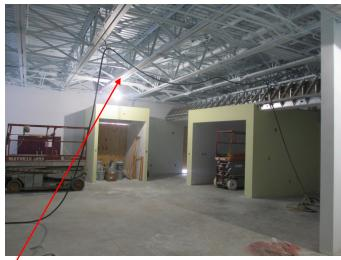
The top-left photo shows the progress of the finishing of the interior of the addition. All of the roof structure and associated mechanical and electrical has been painted white. Some of the wallboard has even been painted.
