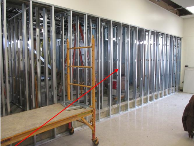
The top-left photo highlights the new double-stud wall that will separate the addition from the existing building. This wall will be filled with insulation in order to acoustically protect the end classroom from noise being generated in the addition.
