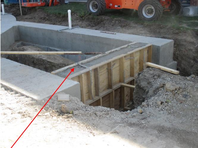
The top-left photo shows another portion of the foundation system being completed. Here the part of the foundation that forms the frost-proof stoop for the new addition entry has been formed and the concrete placed.
