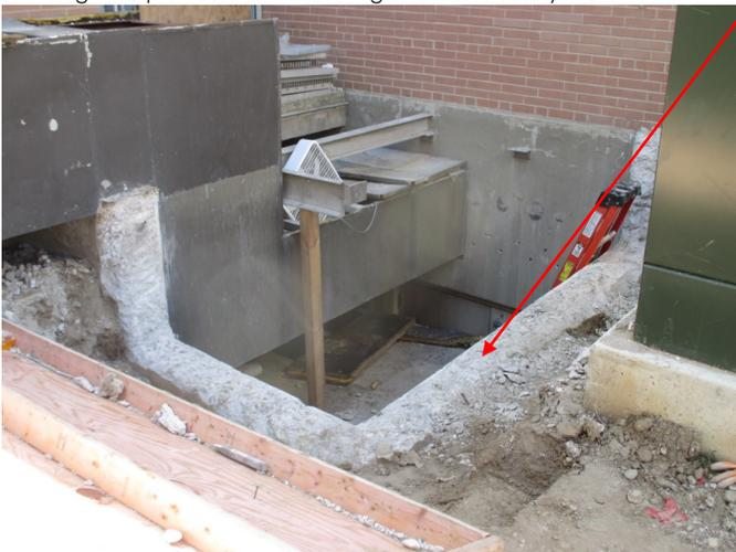
The bottom-left photo shows the beginning of the process to repair the concrete walls of the mechanical pit at the northeast corner of the building. The previous wall was failing and was a safety issue.
