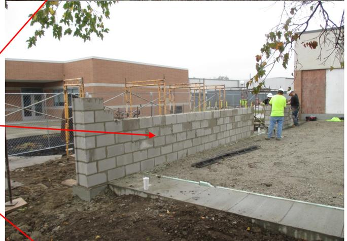
The middle-right photo shows the masons beginning installing the concrete block portion of the north wall of the addition.
