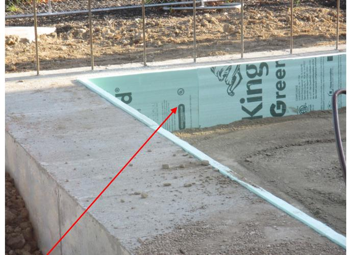
The top-right photo is a close-up highlighting the installation of the rigid insulation board around the perimeter of the foundation.
