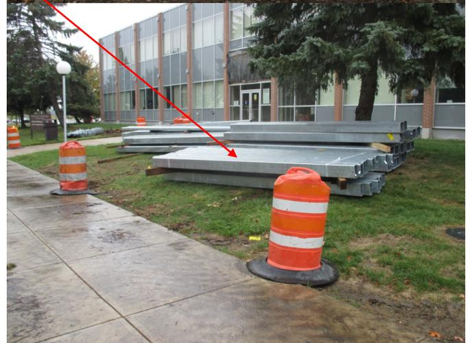
The bottom-right photo shows the one of many stockpiles of steel that was delivered this week and will form the backer system for the sunshades on the south side of the building. This steel will start to be installed next week.
