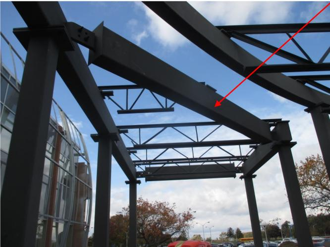
Bar joist sitting on a bearing plate that has studs on the bottom of it that are embedded in the grouted block below and welded in place.
