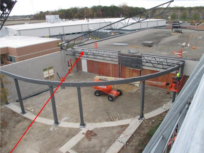
The top-left photo shows the progress of the installation of the open-web bar joists that will support the roof for the addition. You will notice that the bar joists rest on either the new concrete block wall or the new support steel that way they don't add any load to the existing building which might cause damage.
