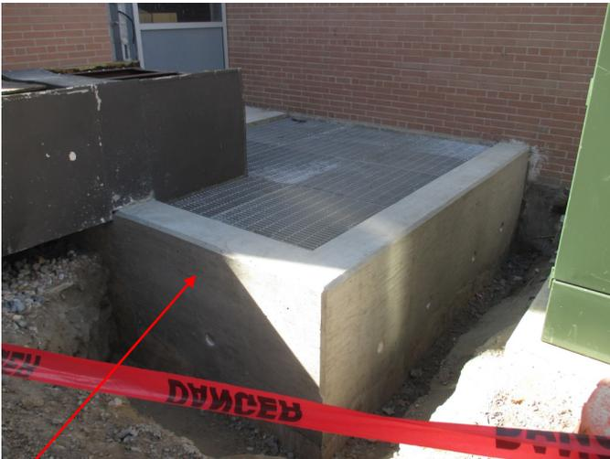
The top-left photo shows the now completed repairs to the mechanical area well concrete walls. The forms have been stripped and the metal grates have been set back in place.
