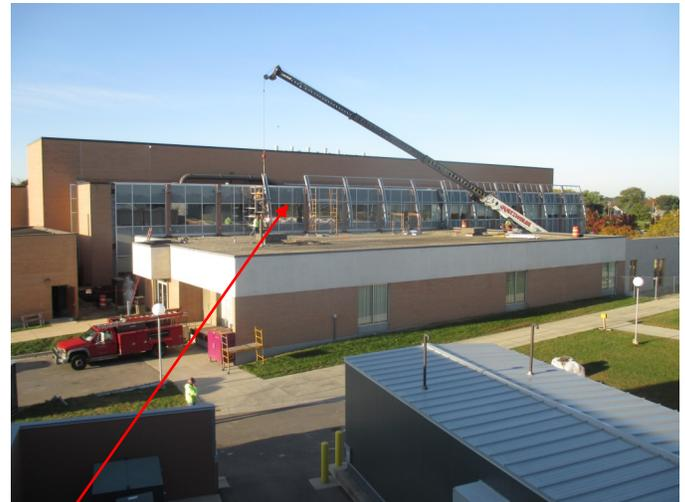
The top-right photo gives a good glimpse of the overall progress of the installation of the support steel being erected on the north face of the building for the new shade system. Only a few bays are left to receive steel, and then in a few weeks the mesh panels will be installed.
