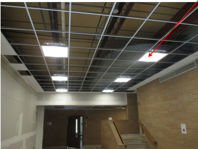
The bottom-left photo shows the progress of the installation of the new ceiling track and tile as well as the new lighting outside the lecture hall in the existing building. The new LED lighting in this area is not only much more energy efficient, but brighter.
