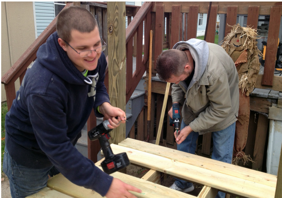
Dean Kerste, professor of mechanical design technology, and a student construct a barrier-free access ramp for a local resident who has multiple sclerosis.
