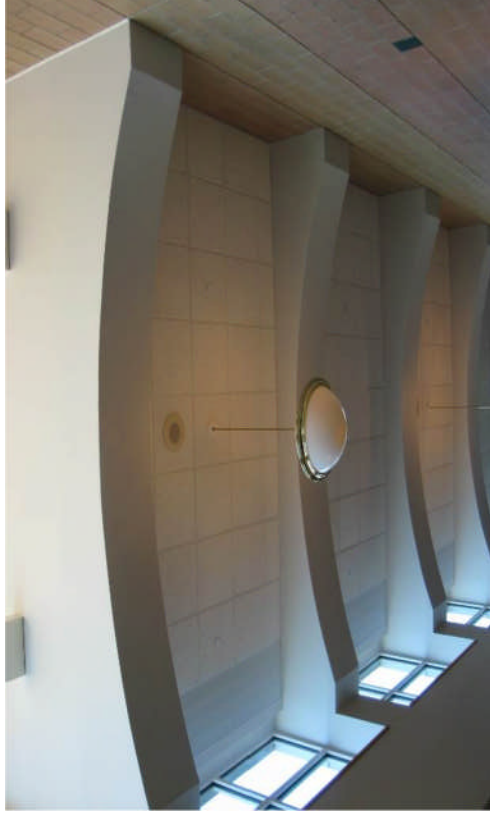
Health Education Building – Daylighting controls for the Atrium would save energy.
